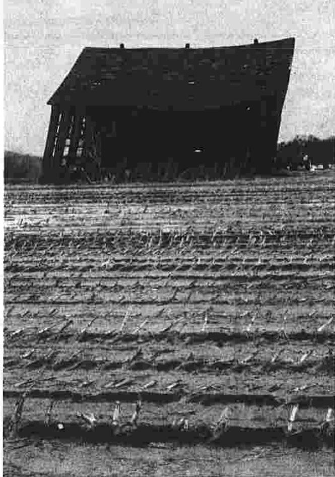
The leaning tobacco shed on Hillstown Rd.
